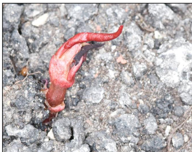
Figure 4 Japanese knotweed is extremely difficult to eradicate and can cause structural damage to roads and houses by growing through asphalt and concrete. This can lead to significant delays and costs to development, estimated at £150 million a year. (Source: GBNNSS)
