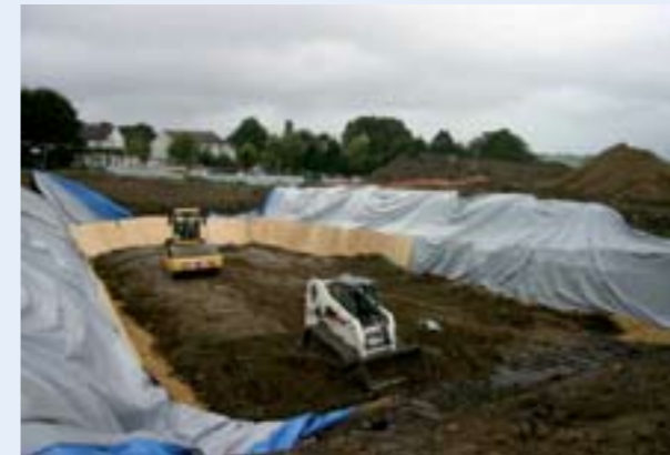
Stage 5: Fill the cell with the knotweed infested soil. No other material, contaminants, or wastes should be included.
