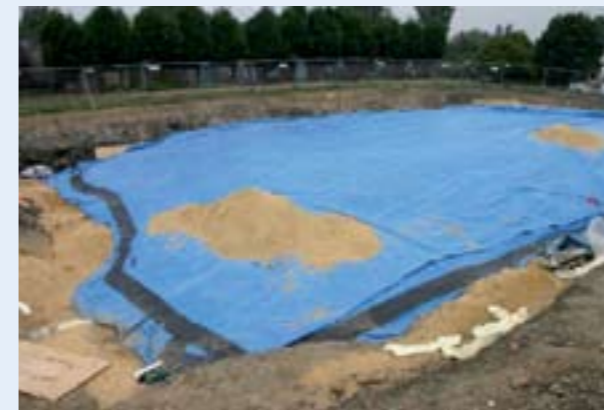
Stage 7: Put the surface of the root barrier membrane in place and make sure the cell is adequately sealed.
