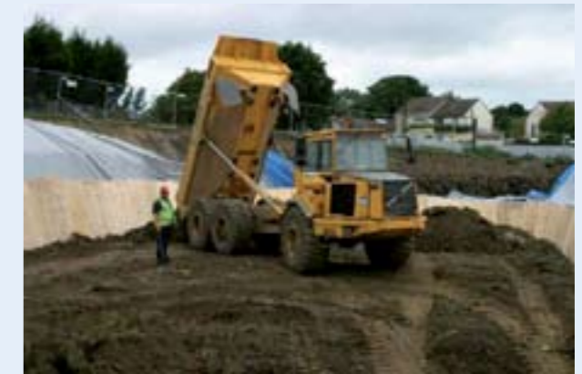
Stage 6: Make sure that dedicated vehicles are used and cleaned properly after they have been used. Haulage routes must be protected.
