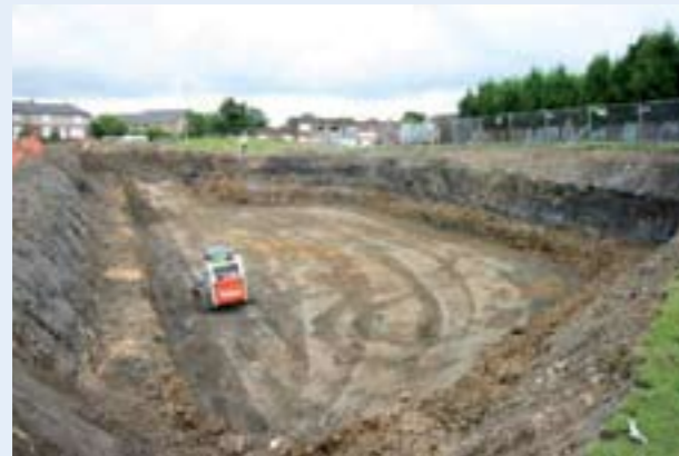
Stage 1: Calculate volume required and excavate site, allowing for 2m depth of burial
