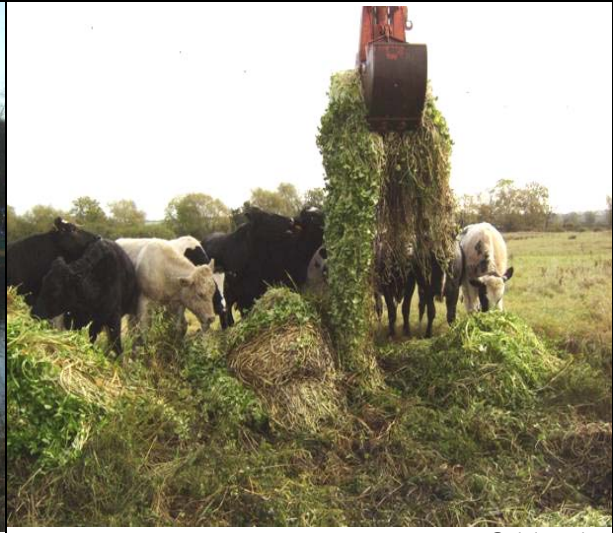
Excavators tend to create large piles of weed, although these rot away within 2 – 3 weeks, the risk of reintroduction to the channel is high
