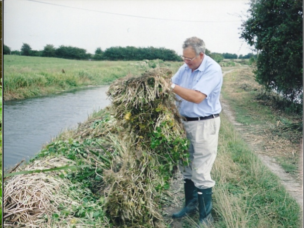
Excavators tend to create large piles of weed, although these rot away within 2 – 3 weeks, the risk of reintroduction to the channel is high
