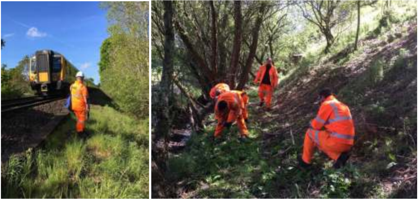
Photos taken by Jo Gore of Network Rail staff along the main line railway at Brockenhurst in the vicinity of the Lymington River on 13 May 2019
